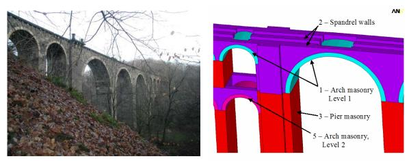
Figure 3: Masonry arch bridge (left), material areas (right)
